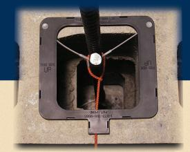
The Rebar-Lok system features a high-impact polystyrene casing that houses a built-in tie wire in the perimeter of the frame. During wall construction, the mason simply mortars the Rebar-Lok into place. Once the desired wall height is reached, the mason places the rebar, then pulls the looped tie wire to engage the system, automatically centering the rebar at the core. He then pours the grout to complete the installation.
